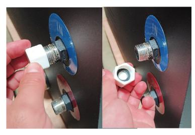
When removing the Caps please be sure that the Gaskets on the inside of the Caps are not left on the Inlet or Outlet Fittings.
