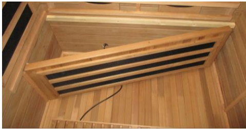
FIG-9 Installing Bench Heater
