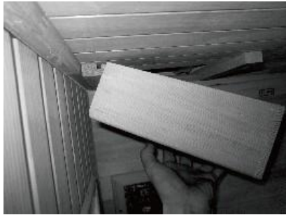
FIG-16 Installing the Radio Wood Housing
