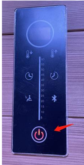
Sauna's Control Panel is OFF (power button is red)
