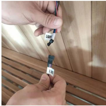
Rear Wall – Middle Light Connection
