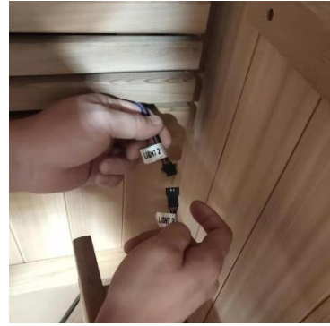
Rear Right – Corner Light Connection
